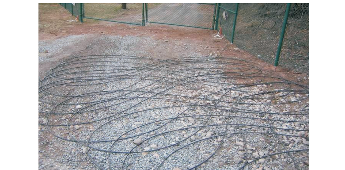
Figure 56 Laying cable in a figure-8 pattern
