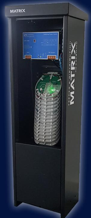
*The InOne Power Rectifier, Power tray and Fiber Trays integrated into Hexatronic MATRIX Compact Fiber Access Terminal*
